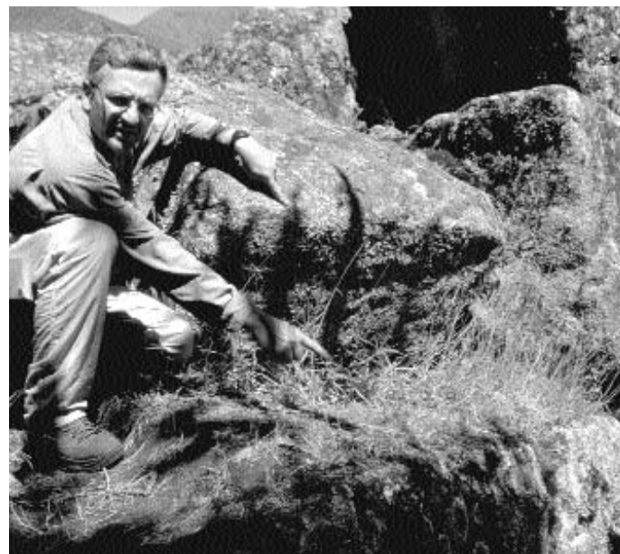
Figure 4. Geologist Eric Bikis points to the underside of a tilted stone at the Unfinished Temple that was in the process of final shaping in AD 1540 so that it would fit snugly onto the stone below. The huge wall was nearly complete when the workers left.
