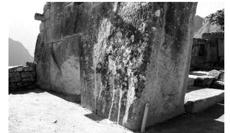
Figure 7. Visitors to Machu Picchu can clearly see the work in progress at the Temple of the Three Windows that was never completed. The supervisor's vertical line on the west side of the building wall and the already finished wall surface show exactly what still remained to be finally shaped.
