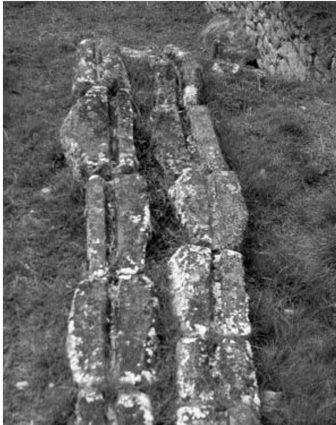
Figure 8. The shape and character of unused channel stones that someday were to carry water to new fountains provides evidence of good civil engineering.
