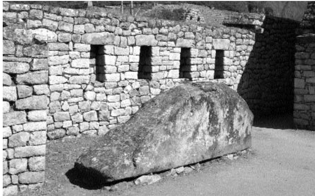
Figure 3. The stone in the eastern Urban Sector was in transit when Machu Picchu was abandoned. It would later have been shaped at its final destination.
